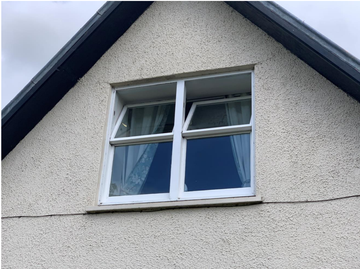
Front Windows (Showing opening style)
