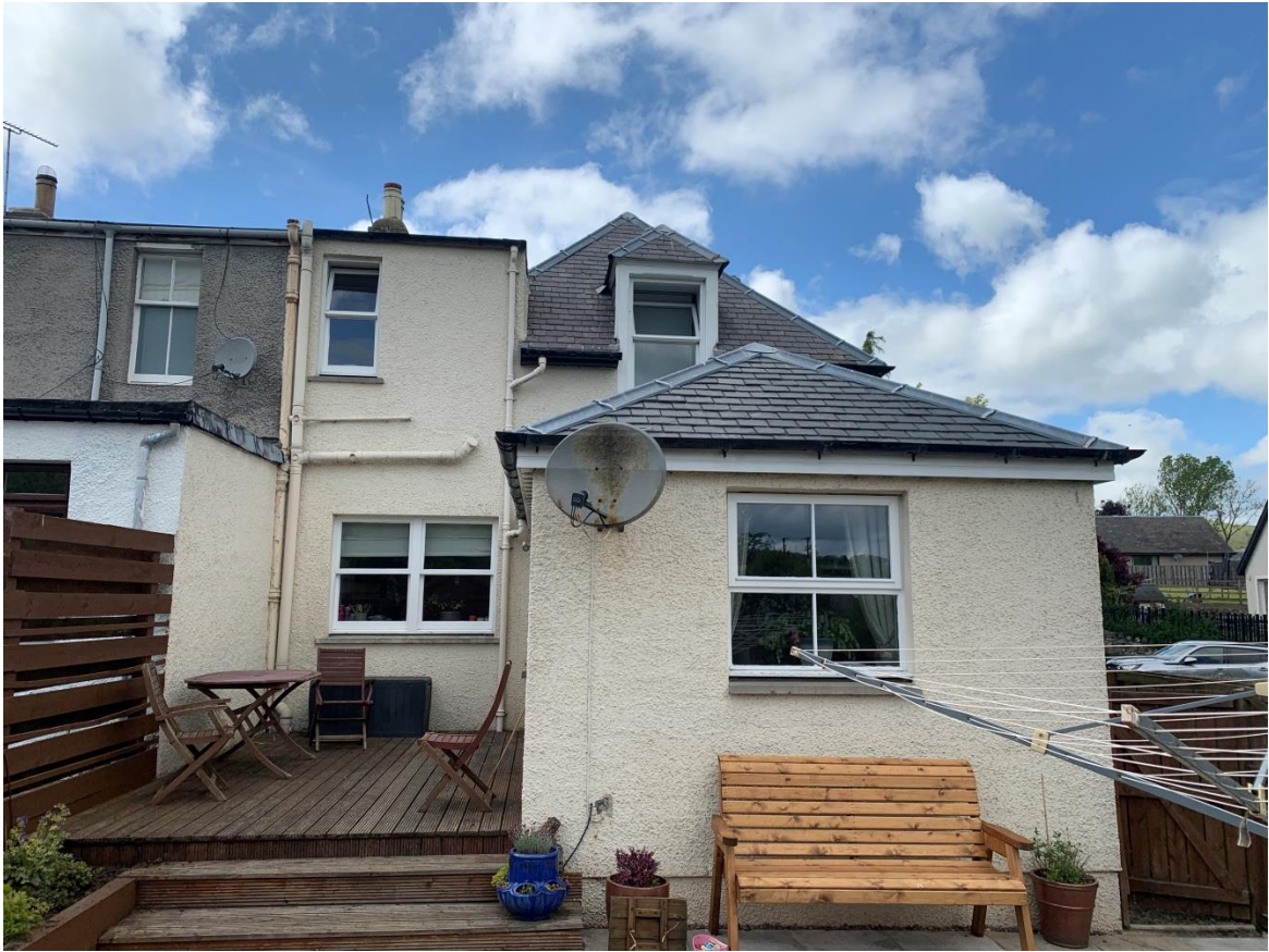
Rear View of House/South-East Elevation
