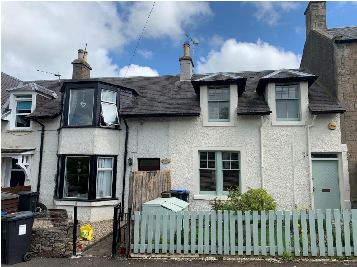
Front Elevation of 'Craiglea' & 'Glenisla' (Aluminium framed casement to Craiglea, Green painted timber vertical sliding to Glenisla)
