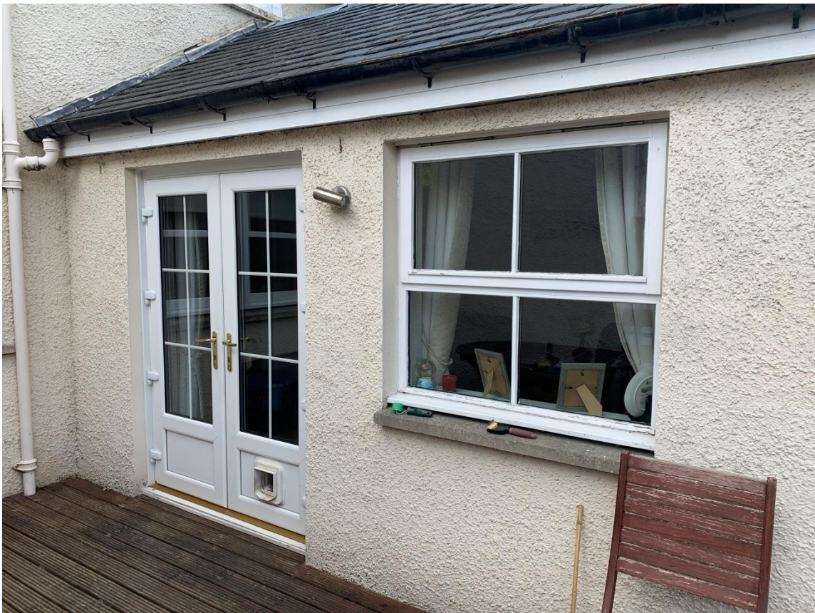
South-West Elevation (Previous extension works)
